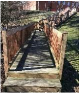
walkway down to Old Road and Brook trails
